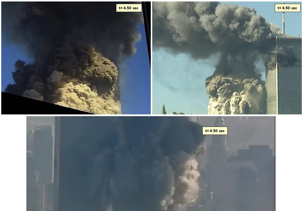
Figure Appendix 19: At t=4.50– The cloud of dust and debris expands with no structure clearly discernable.
