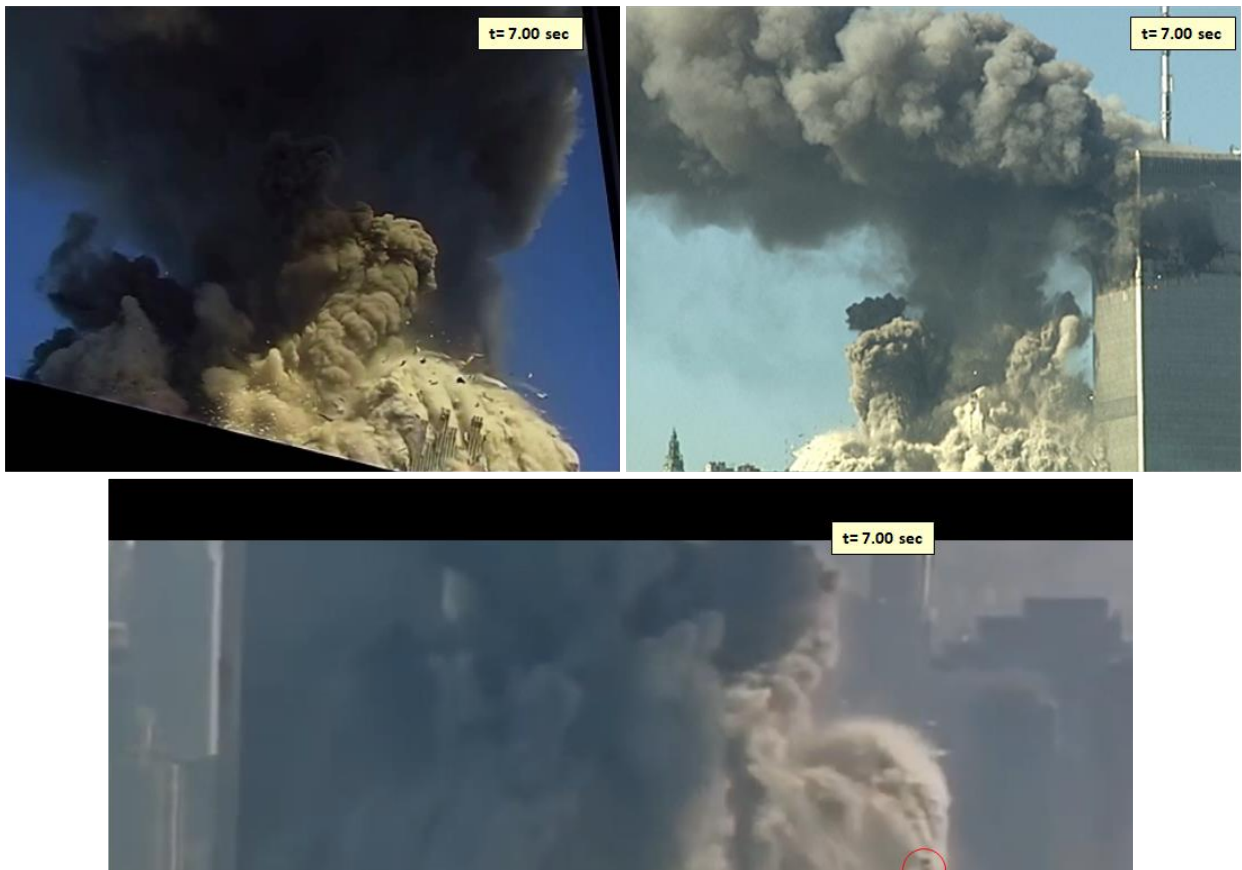
Figure Appendix 29: At t=7.00 – Perimeter columns are clearly seen in the “Reviere” video and descend out-of-sight in the “DeJong” video. These perimeter column sections are captured in the “unnamed” video.
