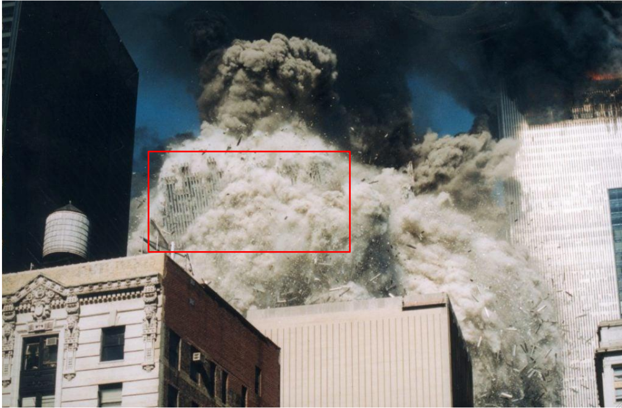
Figure 3: View of the “surfing” perimeter columns, taken nearly perpendicular to its trajectory, shows the width of the wall section which has been ejected as a relatively coherent whole.
