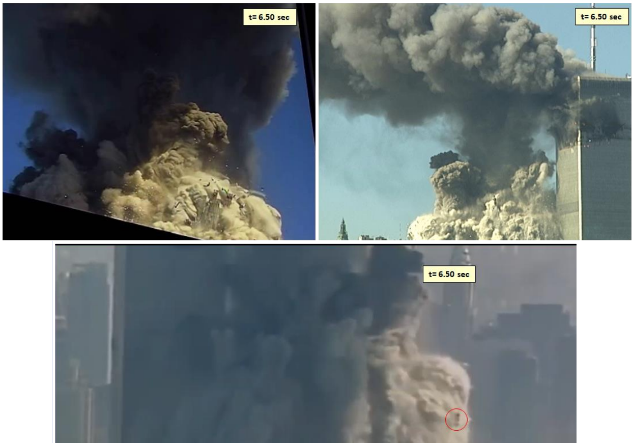
Figure Appendix 27: At t=6.50 – Perimeter columns are clearly seen in the “Reviere” video and in the “DeJong” video. These perimeter column sections are captured in the “unnamed” video.
