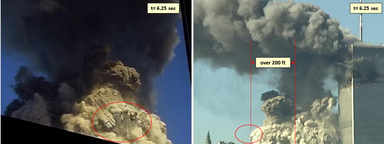
Figure 4: Location of the “surfing” columns from the southeast (left) and the northeast (right) at 6.25 second after the hinging motion begins.
