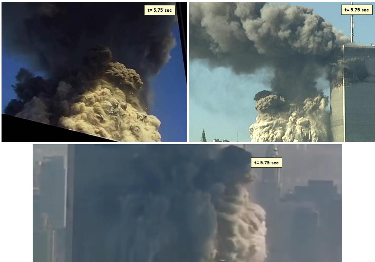
Figure Appendix 24: At t=5.75 sec – Perimeter columns continue to emerge in the “Reviere” video and are clearly seen in the “DeJong” and “unnamed” video.
