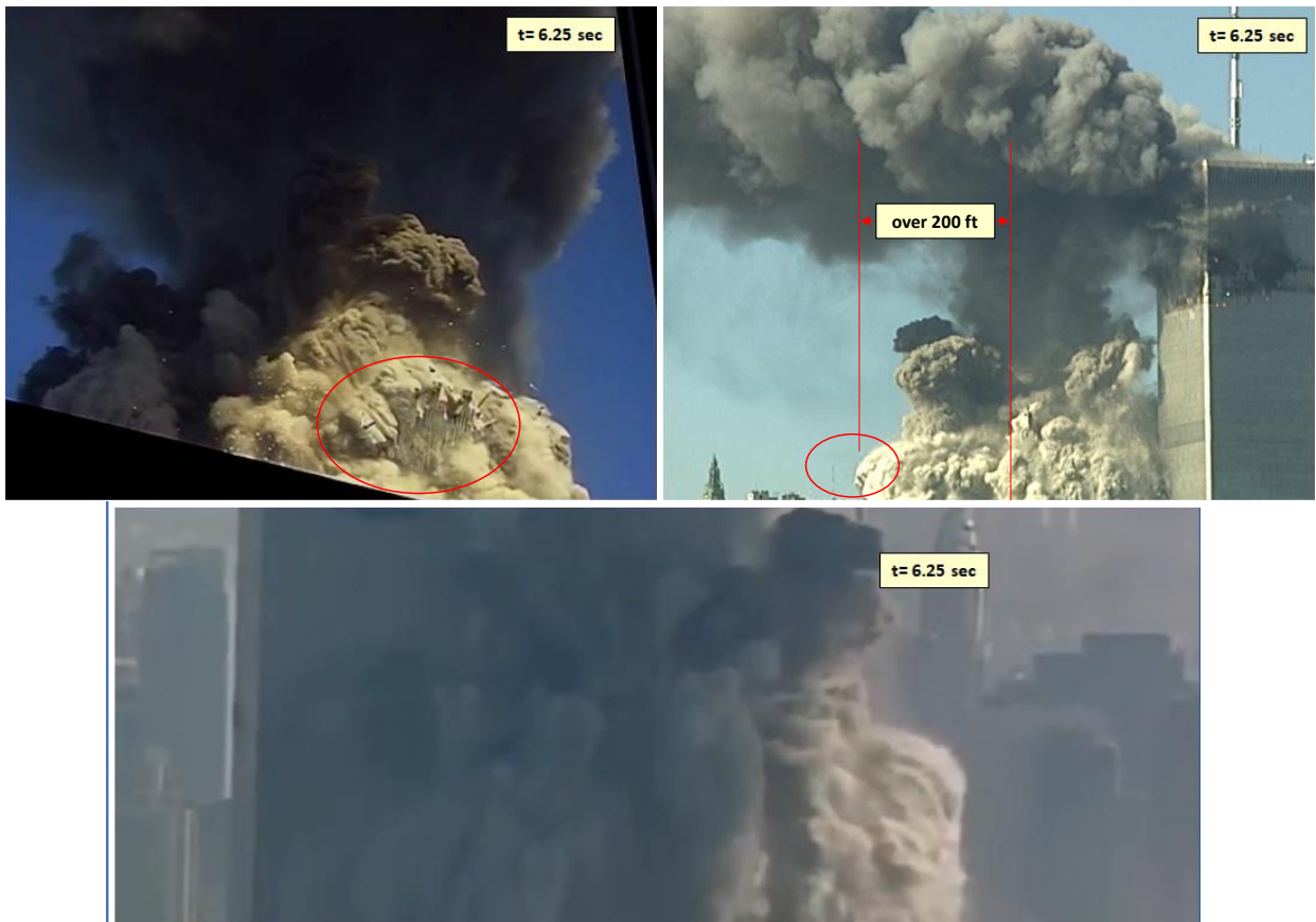
Figure Appendix 26: At t=6.25 sec – Perimeter columns are clearly seen in the “Reviere,” “DeJong” and “unnamed” video. At this point they are over 200 feet from the east side of the Tower.
