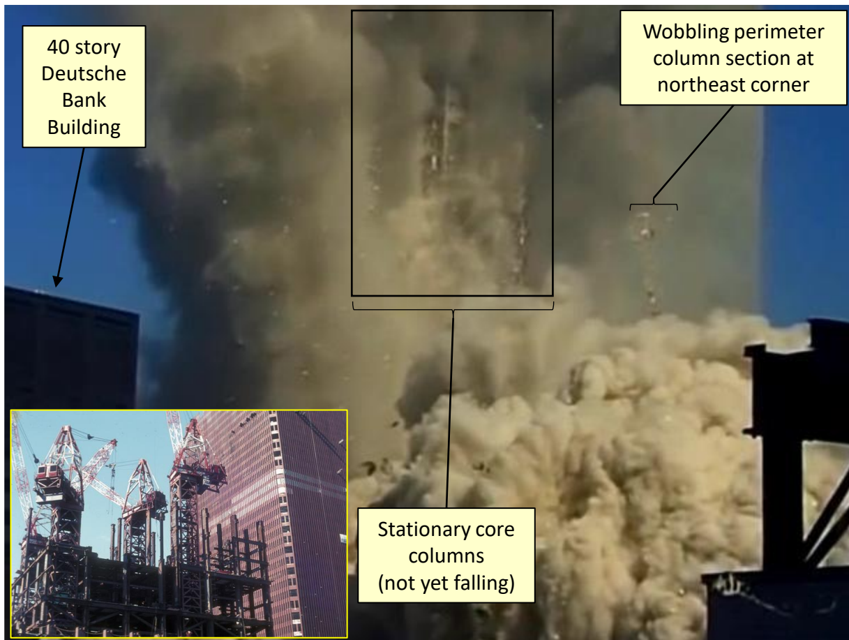
Figure 23: Details of the stationary core columns are seen in the Reviere video once the outer perimeter columns and floor trusses have been propelled away. Inset photo shows the South Tower core during construction from a similar perspective.
